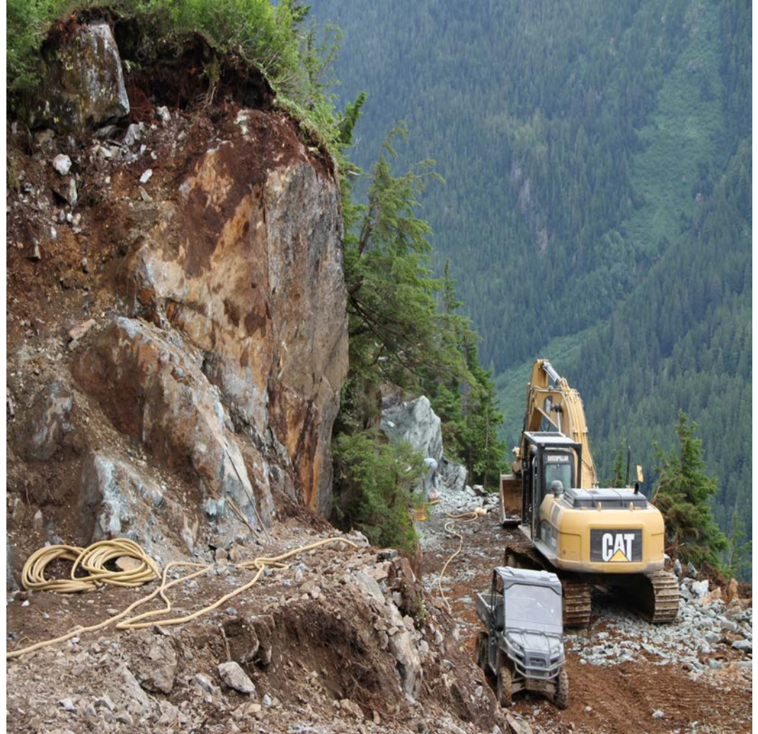
Excavator Trench at North End of Upper Montrose zone.
