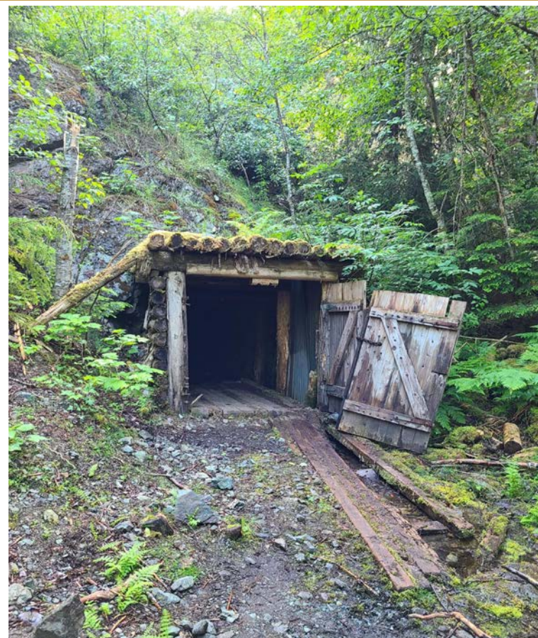
Dardanelle Adit Entrance.
